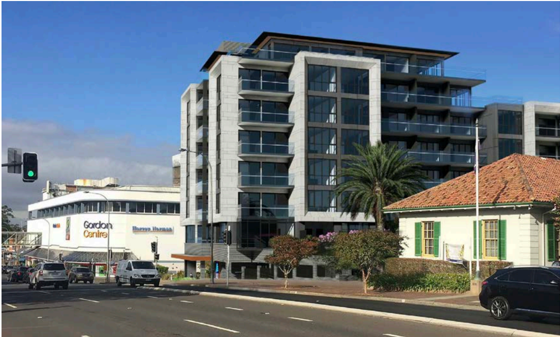
Figure 5: Excerpt DA28 (B) Photomontage – unsatisfactory street activation resulting from supermarket floor level below ground, lack of presence or definition of residential entry, and clear residential dominance in the primary streetscape
